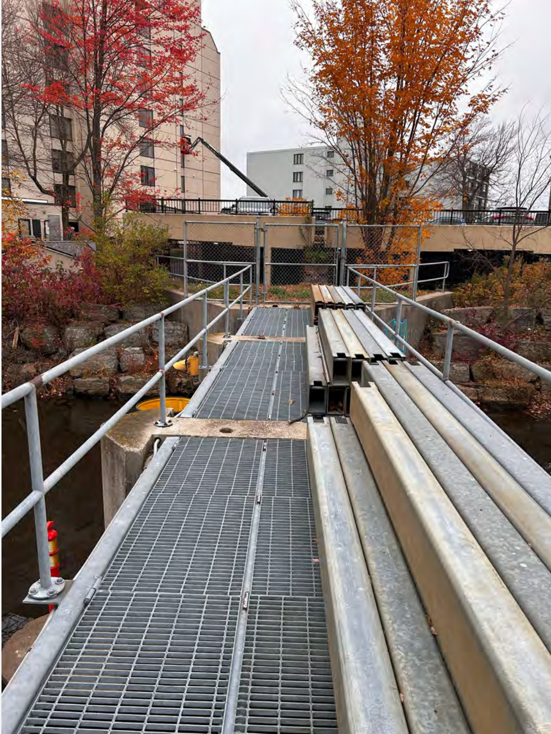
Galvanized Metal Deck, Supports and Barrier Railings
