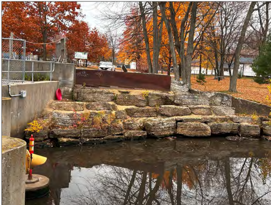
Concrete Outfall Structure
