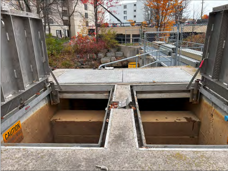
Concrete Pump Chamber
