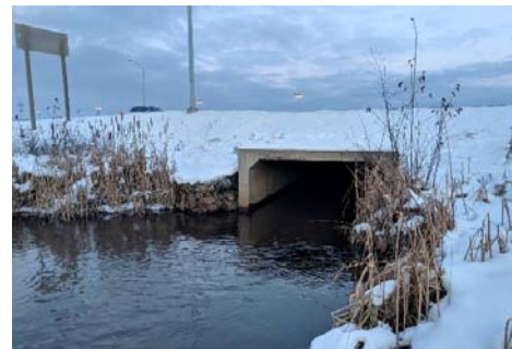
Description: Looking at d/s face
