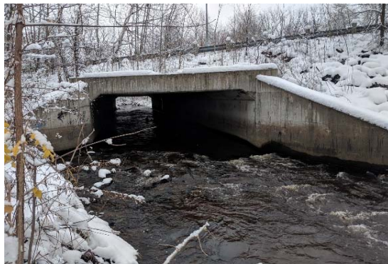
Description: Looking at d/s face
