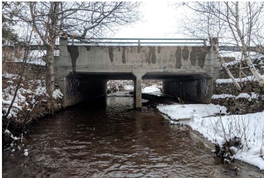
Description: Looking at d/s face
