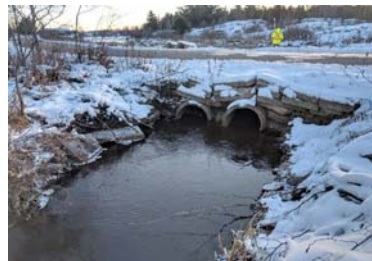
Description: Looking at d/s face
