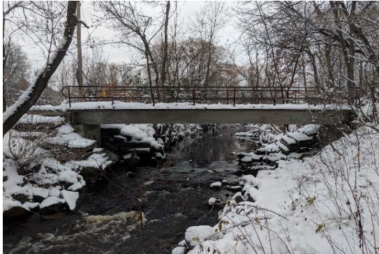
Description: Looking at d/s face
