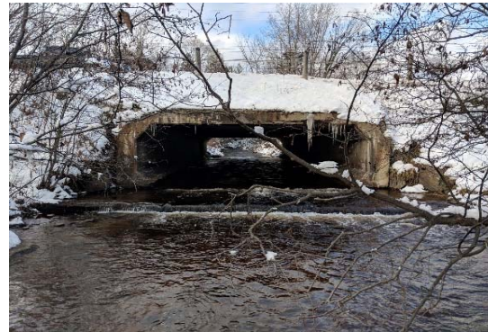
Description: Looking at d/s face
