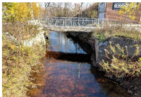
Description: Looking at d/s face
