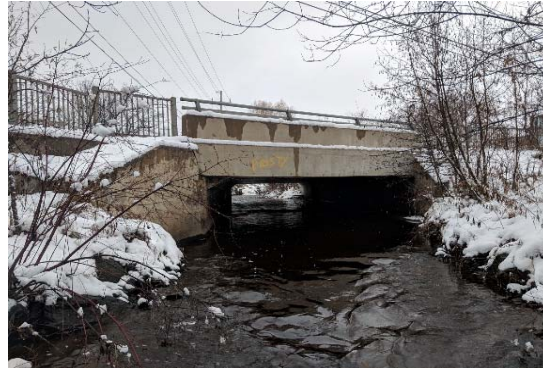
Description: Looking at d/s face
