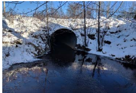
Description: Looking at d/s face
