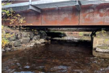
Description: Looking at d/s face
