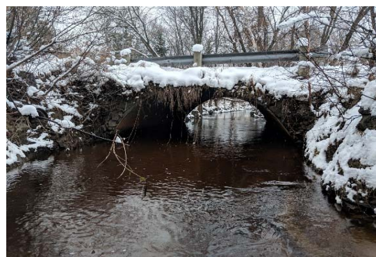
Description: Looking at d/s face
