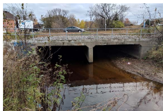
Description: Looking at d/s face
