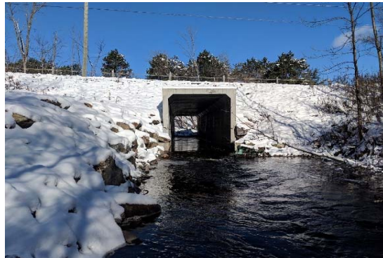
Description: Looking at d/s face
