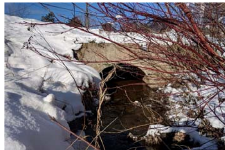
Description: Looking at d/s face
