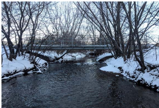
Description: Looking at d/s face
