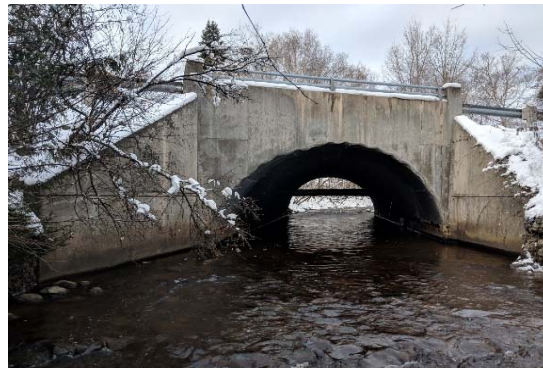
Description: Looking at d/s face
