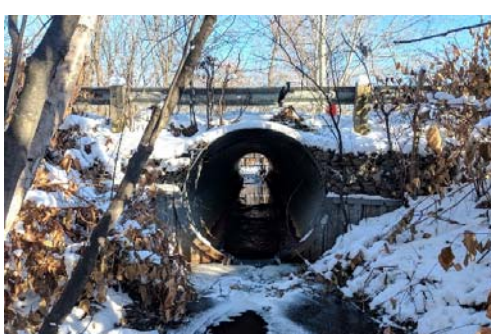
Description: Looking at d/s face
