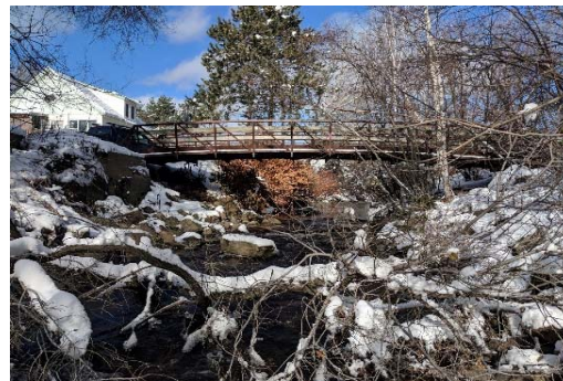
Description: Looking at d/s face
