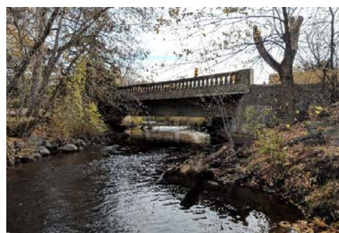
Description: Looking at d/s face
