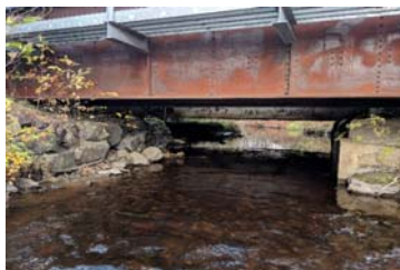
Description: Looking at d/s face
