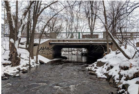
Description: Looking at d/s face
