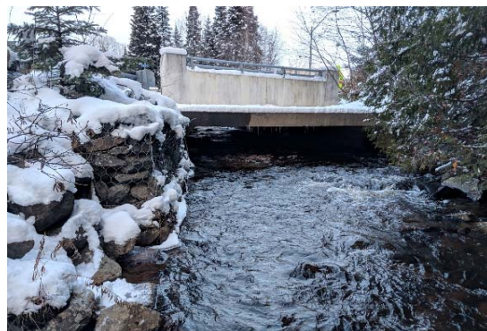
Description: Looking at d/s face
