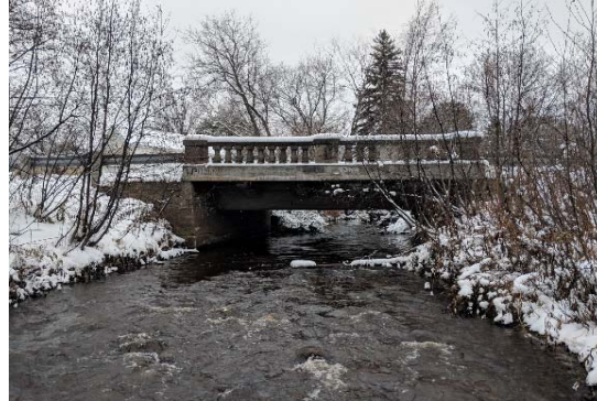
Description: Looking at d/s face
