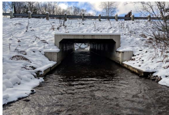
Description: Looking at d/s face
