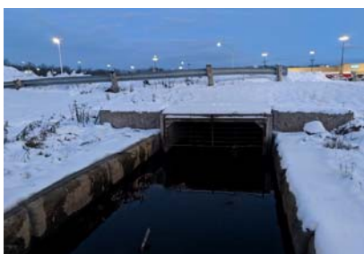
Description: Looking at d/s face
