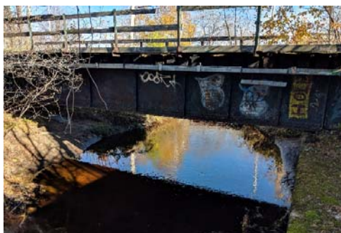
Description: Looking at d/s face
