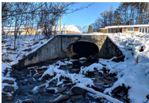
Description: Looking at d/s face
