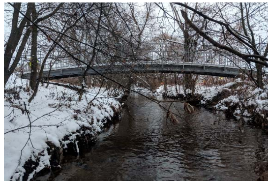
Description: Looking at d/s face
