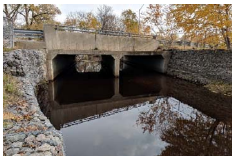
Description: Looking at d/s face
