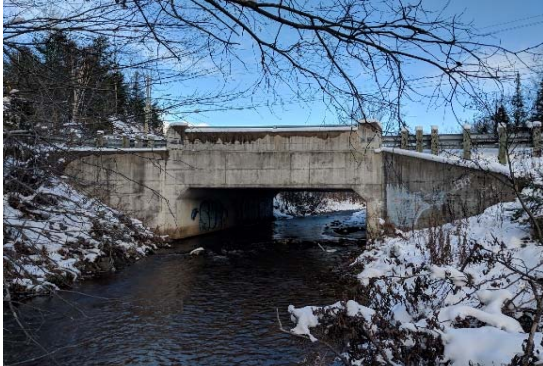
Description: Looking at d/s face
