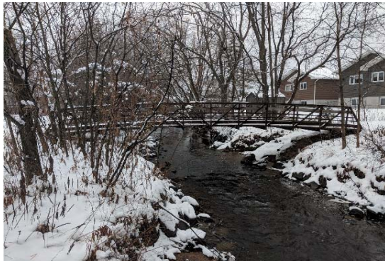
Description: Looking at d/s face
