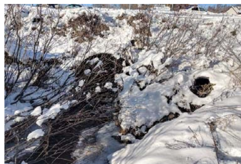
Description: Looking at d/s face
