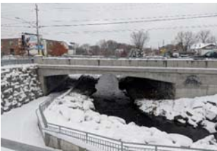
Description: Looking at d/s face
