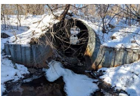
Description: Looking at d/s face
