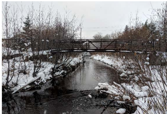
Description: Looking at d/s face
