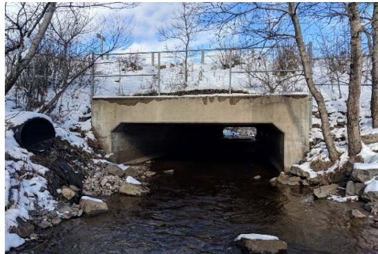
Description: Looking at d/s face
