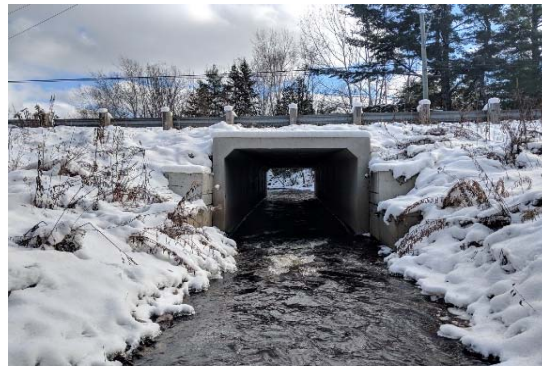
Description: Looking at d/s face
