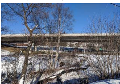
Description: Looking at d/s face
