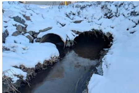
Description: Looking at d/s face
