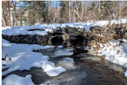
Description: Looking at d/s face
