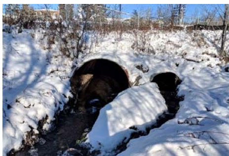
Description: Looking at d/s face
