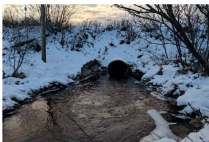
Description: Looking at d/s face
