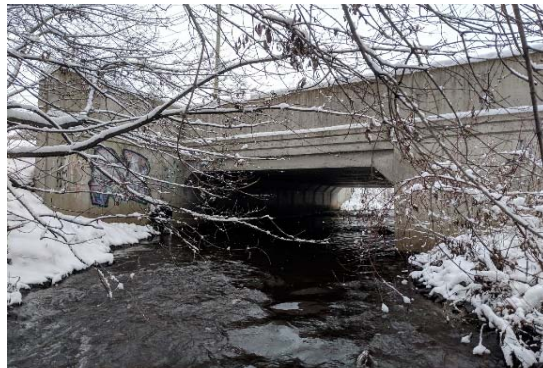
Description: Looking at d/s face
