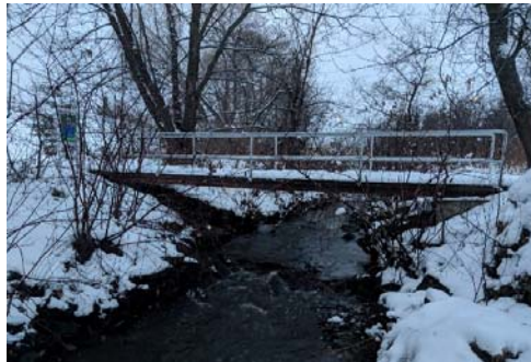
Description: Looking at d/s face
