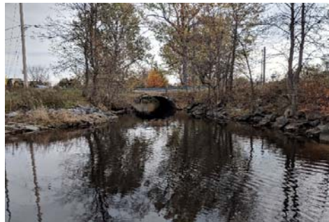
Description: Looking at d/s face
