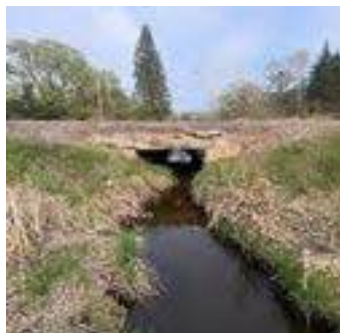
Description: Looking at d/s face
