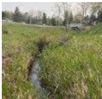
Description: Looking d/s
