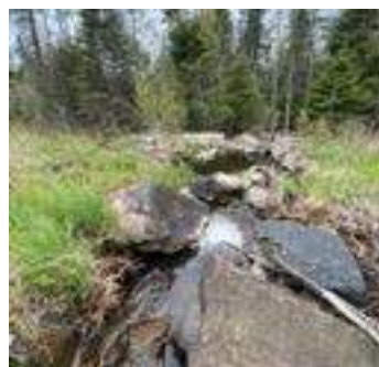
Description: Looking d/s
