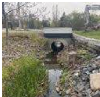
Description: Looking at u/s face
