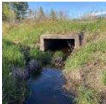
Description: Looking at d/s face
