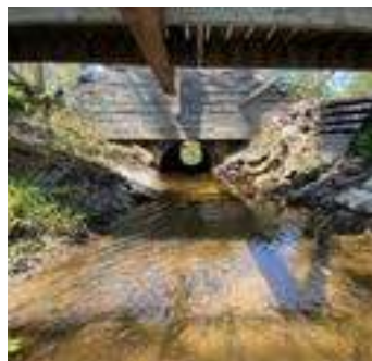
Description: Looking at u/s face
