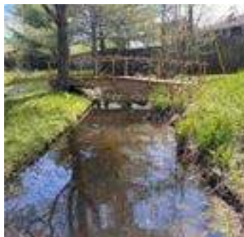
Description: Looking u/s
