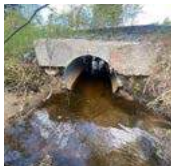
Description: Looking at d/s face
