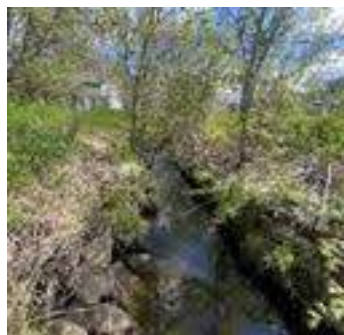
Description: Looking u/s
