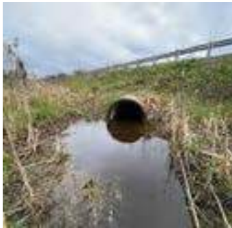
Description: Looking at d/s face
