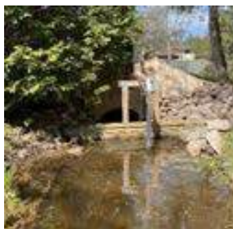
Description: Looking at u/s face
