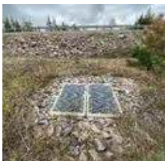
Description: Looking at d/s face
