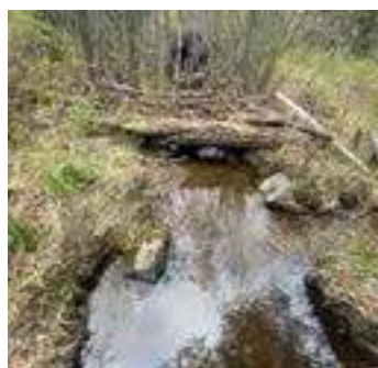
Description: Looking d/s
