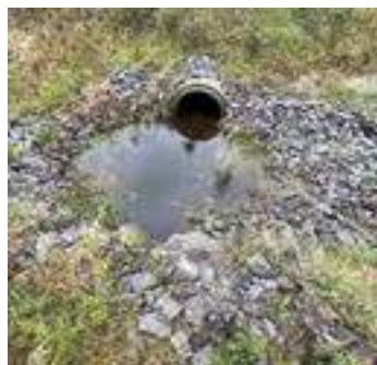
Description: Looking u/s
