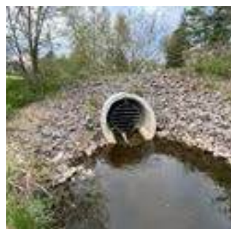
Description: Looking at d/s face
