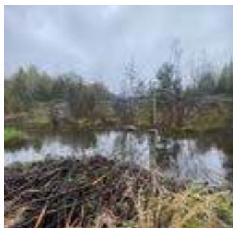
Description: Looking at d/s face
