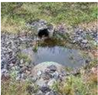
Description: Looking d/s
