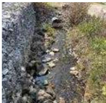
Description: Looking d/s
