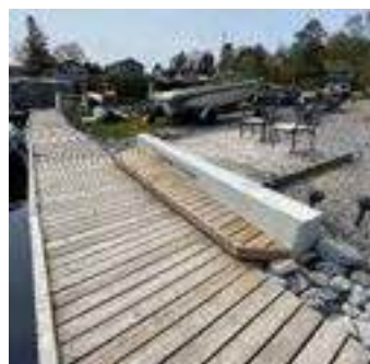
Description: Looking at d/s face
