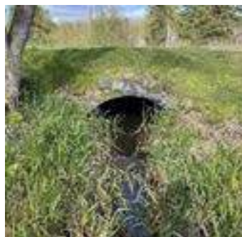
Description: Looking at d/s face
