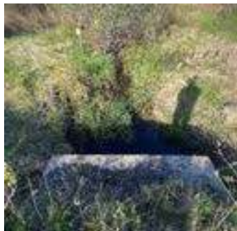
Description: Looking u/s
