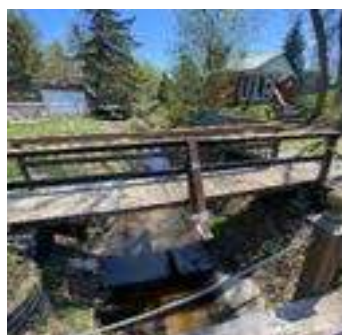
Description: Looking at d/s face
