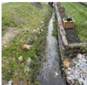
Description: Looking d/s
