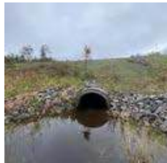
Description: Looking at d/s face
