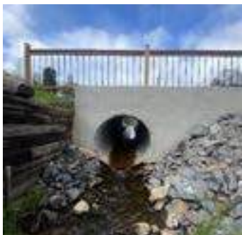
Description: Looking at d/s face
