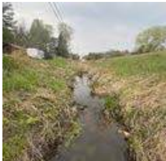
Description: Looking u/s
