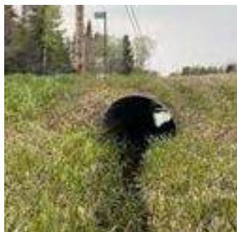
Description: Looking at d/s face
