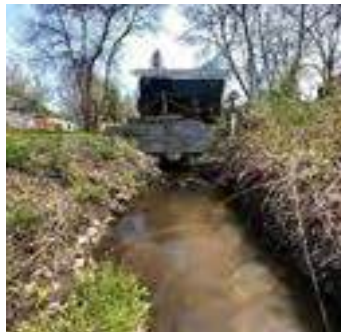
Description: Looking at d/s face
