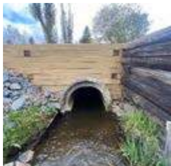
Description: Looking d/s
