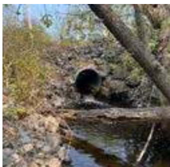
Description: Looking at d/s face
