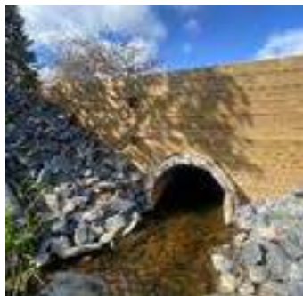
Description: Looking at d/s face
