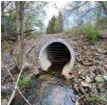
Description: Looking at d/s face
