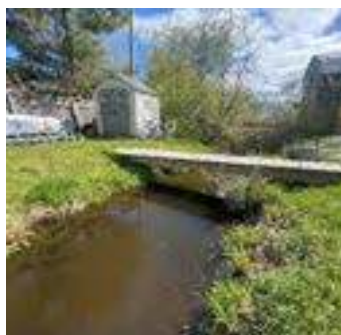
Description: Looking at d/s face
