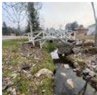
Description: Looking at u/s face
