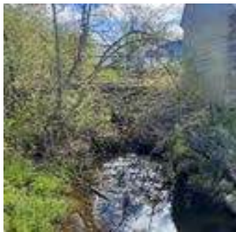
Description: Looking at d/s face
