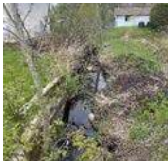
Description: Looking d/s
