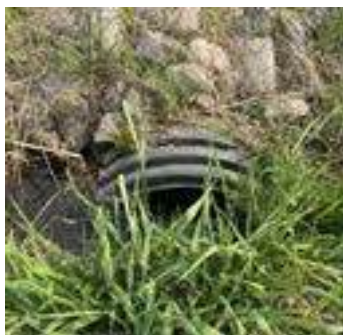
Description: Looking at d/s face
