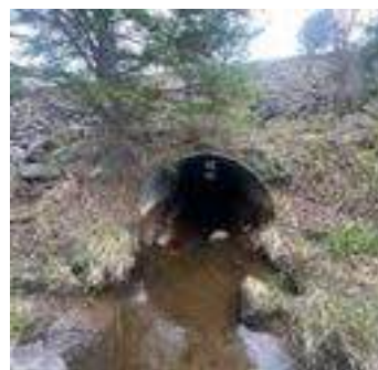
Description: Looking at d/s face
