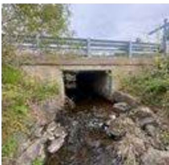
Description: Looking at d/s face
