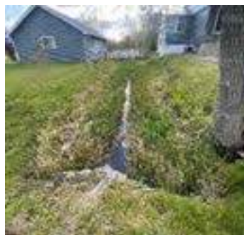
Description: Looking d/s
