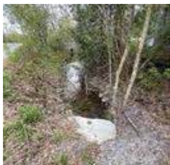
Description: Looking d/s
