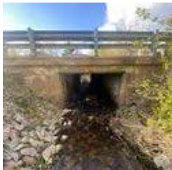
Description: Looking at u/s face
