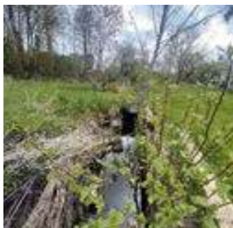
Description: Looking at d/s face
