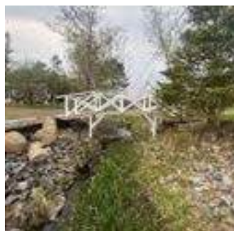
Description: Looking at d/s face
