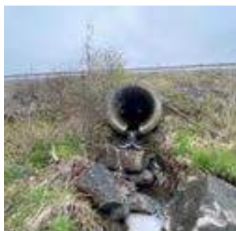
Description: Looking at d/s face
