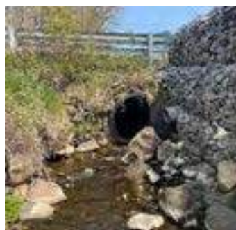
Description: Looking at d/s face
