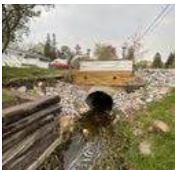
Description: Looking at d/s face
