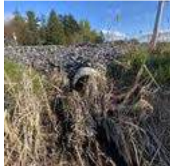
Description: Looking at d/s face
