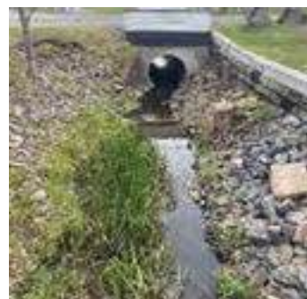
Description: Looking d/s
