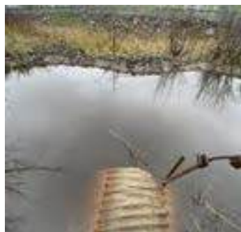
Description: Looking d/s
