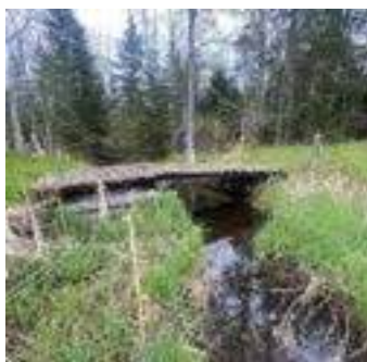
Description: Looking at d/s face
