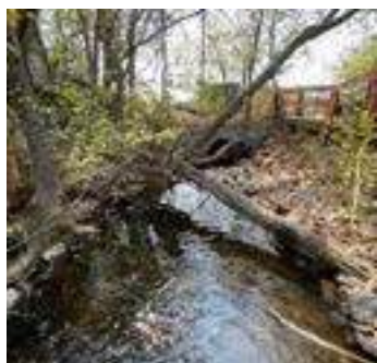
Description: Looking d/s
