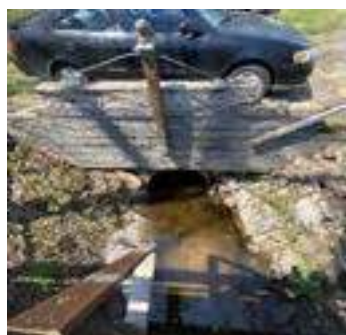
Description: Looking d/s
