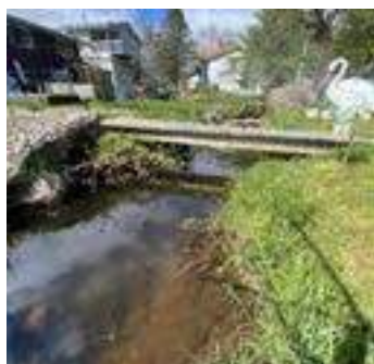
Description: Looking d/s
