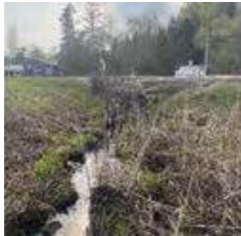
Description: Looking at u/s face
