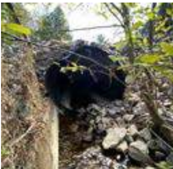
Description: Looking at d/s face
