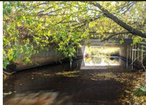
Description: Looking at u/s face
