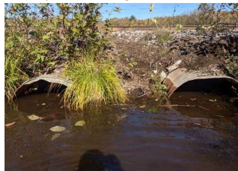
Description: Looking at d/s face
