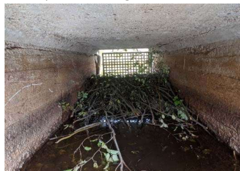
Description: Looking at d/s face
