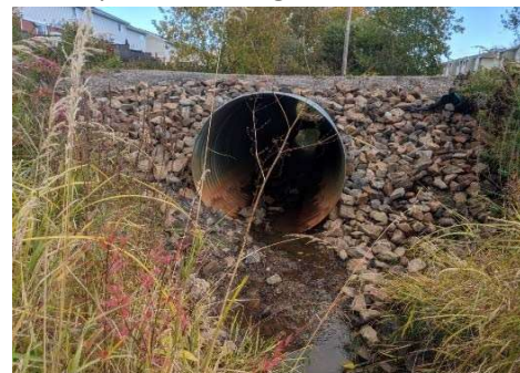
Description: Looking at d/s face
