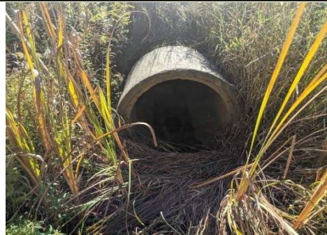
Description: Looking at u/s face
