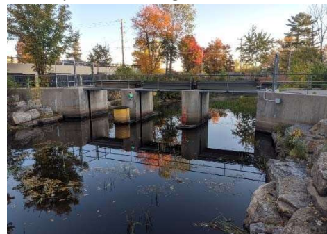
Description: Looking at d/s face
