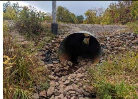
Description: Looking at u/s face
