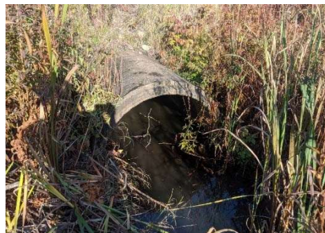
Description: Looking at d/s face
