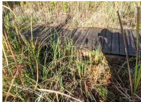
Description: Looking at d/s face
