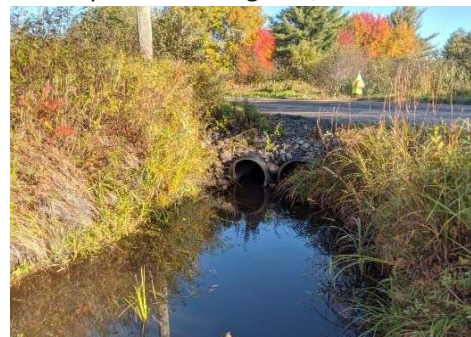
Description: Looking at d/s face
