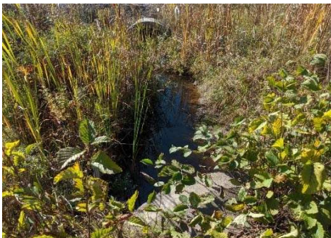
Description: Looking d/s
