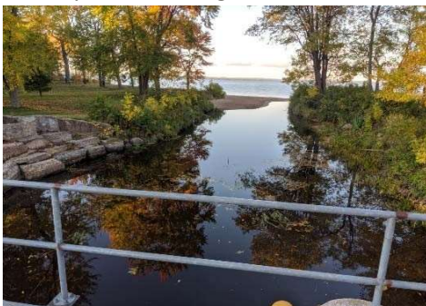
Description: Looking d/s
