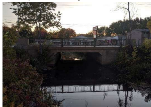
Description: Looking at d/s face
