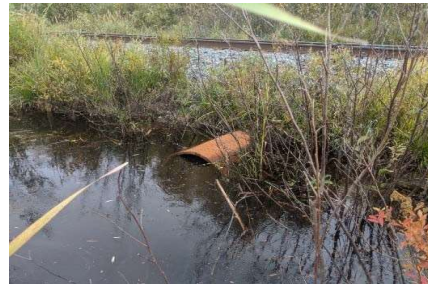
Description: Looking at d/s face
