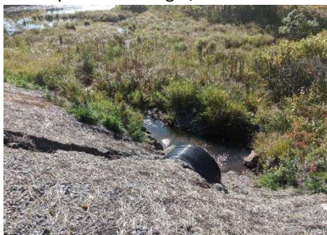
Description: Looking d/s
