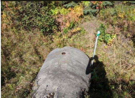
Description: Looking u/s
