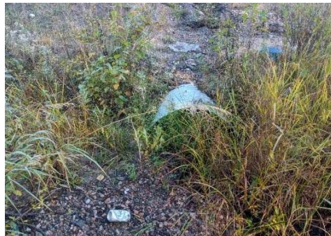
Description: Looking at d/s face
