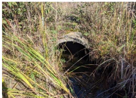
Description: Looking at d/s face
