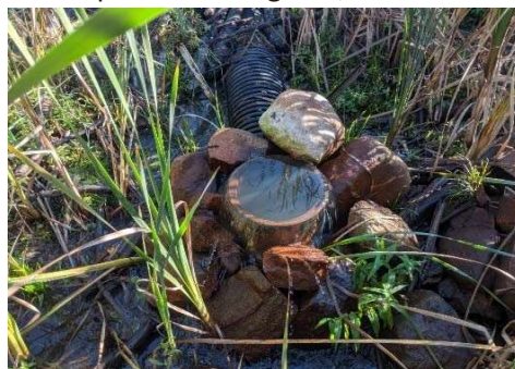
Description: Looking at d/s face
