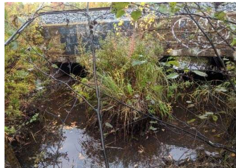
Description: Looking at d/s face
