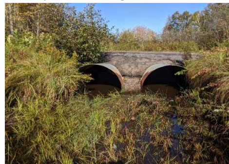
Description: Looking at d/s face
