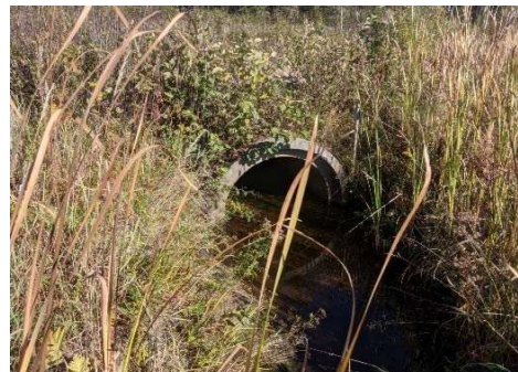
Description: Looking at d/s face
