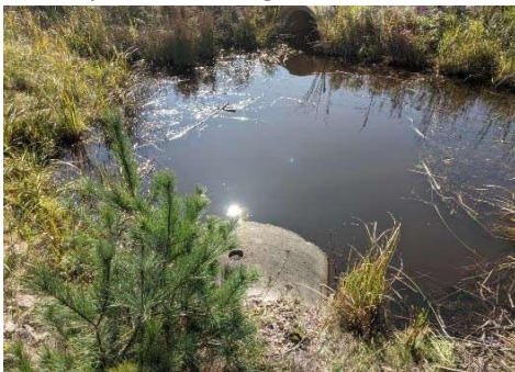
Description: Looking d/s
