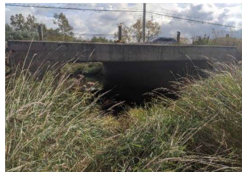
Description: Looking at d/s face
