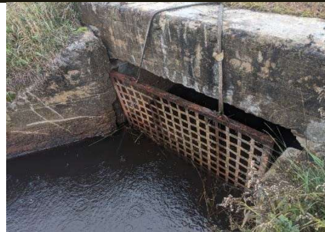
Description: Looking at u/s face
