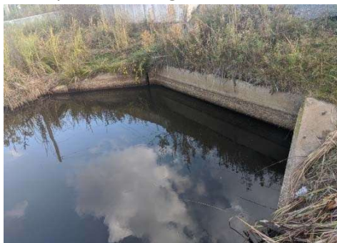
Description: Looking at d/s face
