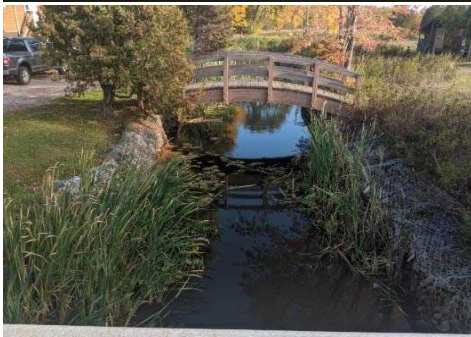
Description: Looking u/s
