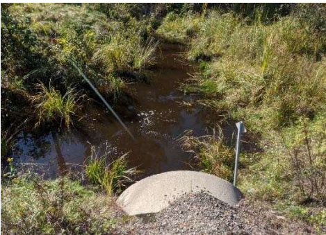
Description: Looking d/s
