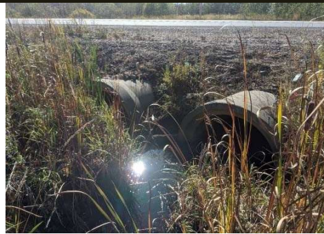
Description: Looking at u/s face
