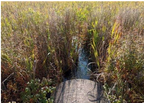
Description: Looking d/s
