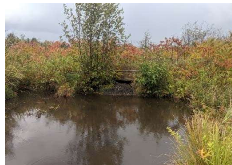
Description: Looking at d/s face
