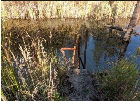
Description: Looking u/s
