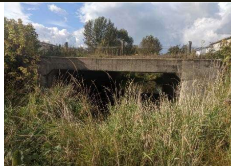
Description: Looking at u/s face
