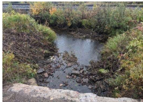
Description: Looking d/s
