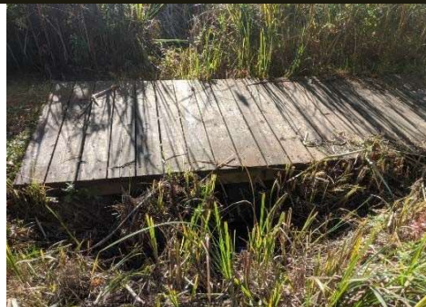
Description: Looking at u/s face
