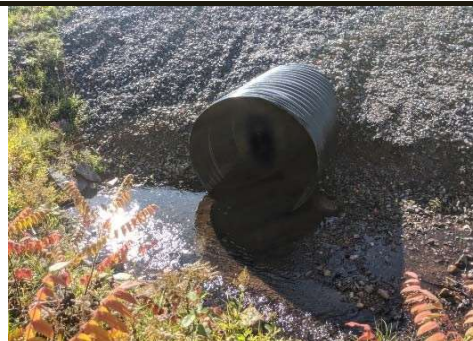
Description: Looking at u/s face
