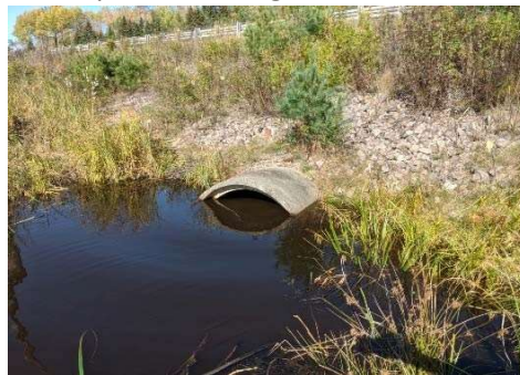
Description: Looking at d/s face
