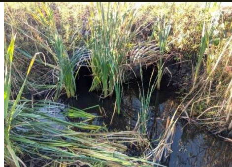
Description: Looking at u/s face
