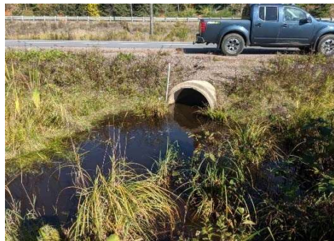
Description: Looking at d/s face
