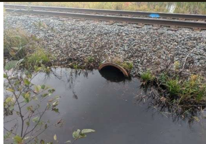
Description: Looking at u/s face
