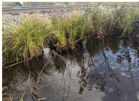
Description: Looking at d/s face
