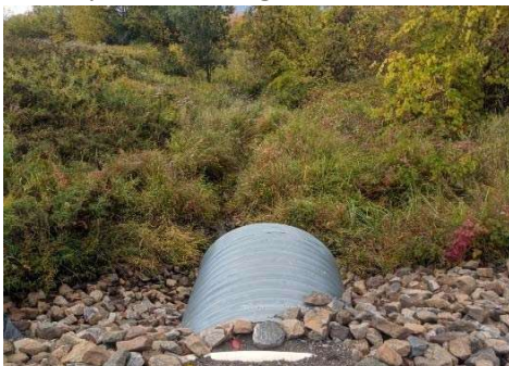
Description: Looking d/s
