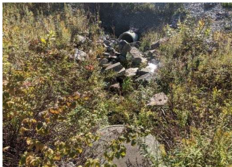
Description: Looking d/s
