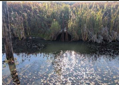
Description: Looking at u/s face
