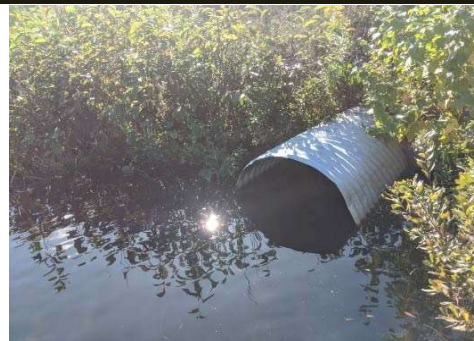
Description: Looking at u/s face
