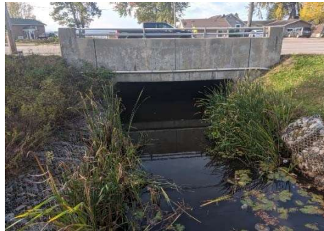
Description: Looking at d/s face
