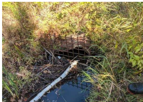
Description: Looking at d/s face
