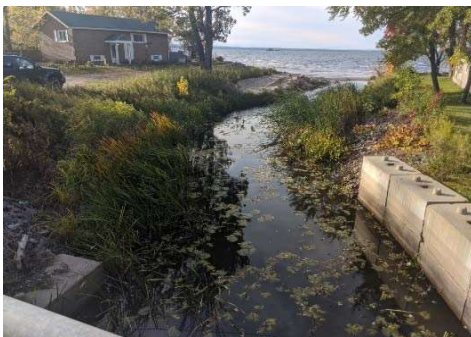
Description: Looking d/s
