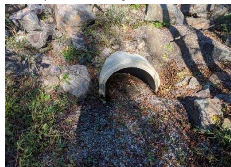
Description: Looking at d/s face
