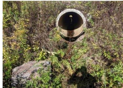
Description: Looking at d/s face
