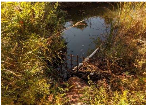
Description: Looking d/s
