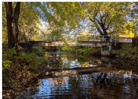
Description: Looking at d/s face
