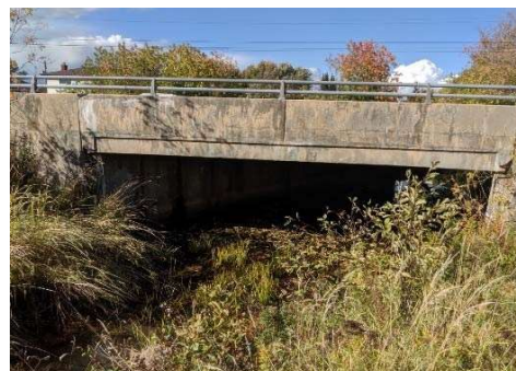
Description: Looking at d/s face
