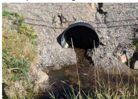
Description: Looking at d/s face
