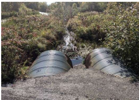
Description: Looking d/s
