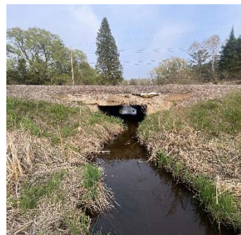
Description: Looking at d/s face
