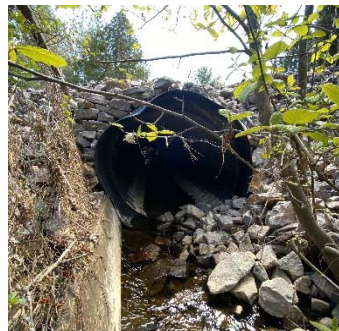
Description: Looking at d/s face
