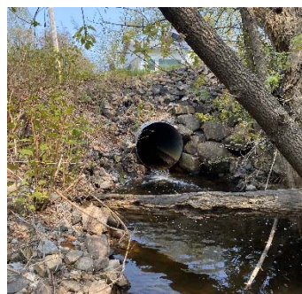
Description: Looking at d/s face
