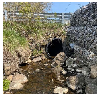
Description: Looking at d/s face
