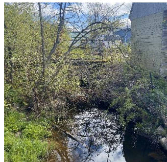
Description: Looking at d/s face
