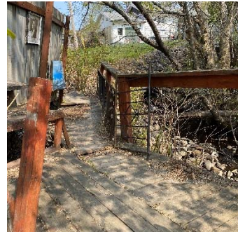
Description: deck on right bank
