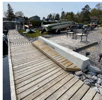
Description: Looking at d/s face
