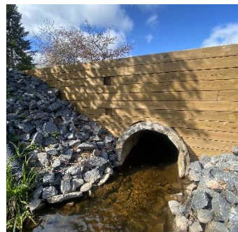
Description: Looking at d/s face
