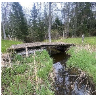
Description: Looking at d/s face
