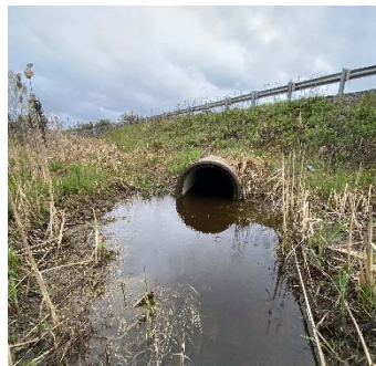
Description: Looking at d/s face
