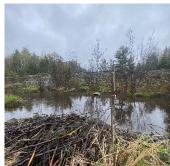
Description: Looking at d/s face
