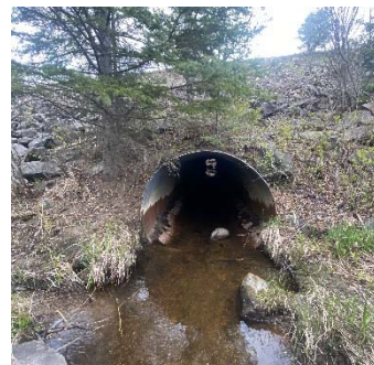
Description: Looking at d/s face
