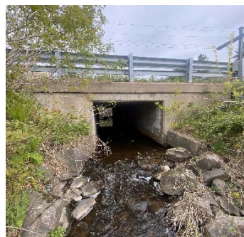
Description: Looking at d/s face
