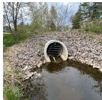
Description: Looking at d/s face
