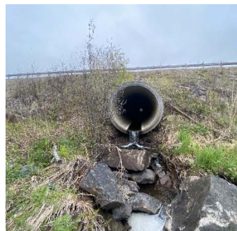
Description: Looking at d/s face
