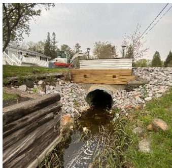
Description: Looking at d/s face
