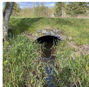
Description: Looking at d/s face
