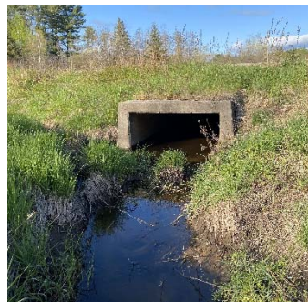
Description: Looking at d/s face
