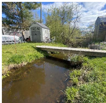
Description: Looking at d/s face
