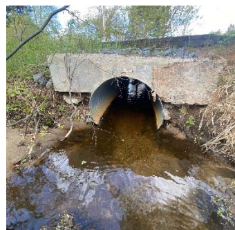
Description: Looking at d/s face
