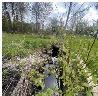
Description: Looking at d/s face
