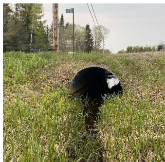
Description: Looking at d/s face
