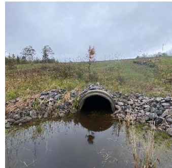
Description: Looking at d/s face
