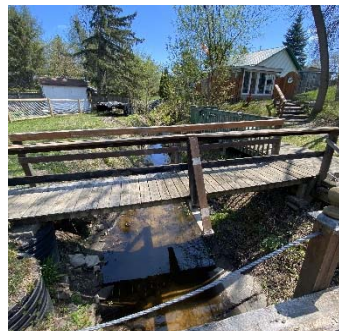
Description: Looking at d/s face
