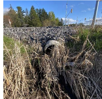
Description: Looking at d/s face
