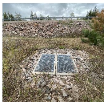
Description: Looking at d/s face
