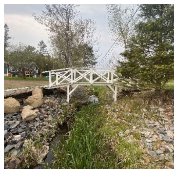
Description: Looking at d/s face
