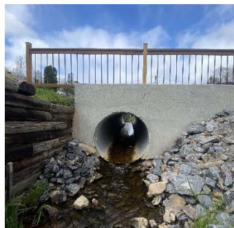
Description: Looking at d/s face
