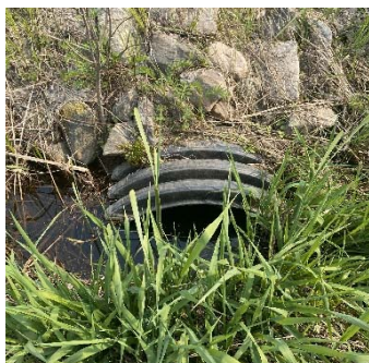
Description: Looking at d/s face
