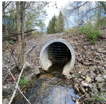
Description: Looking at d/s face
