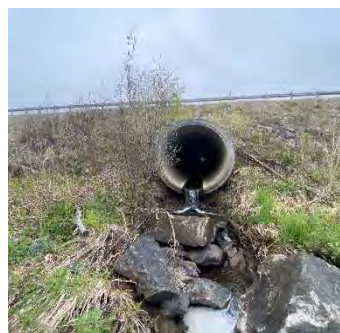
Description: Looking at d/s face
