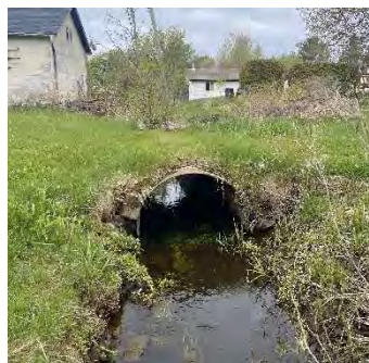
Description: Looking at u/s face
