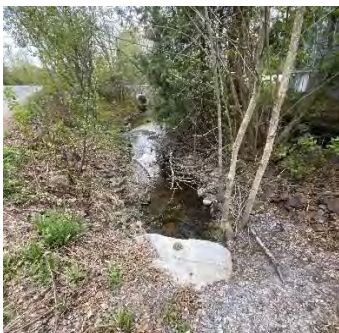
Description: Looking d/s
