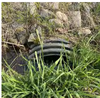
Description: Looking at d/s face
