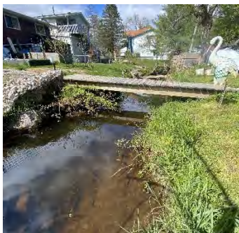
Description: Looking d/s
