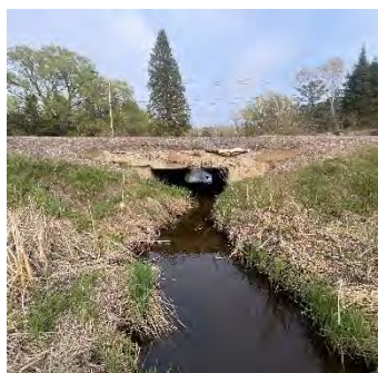
Description: Looking at d/s face
