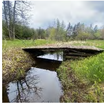
Description: Looking at u/s face
