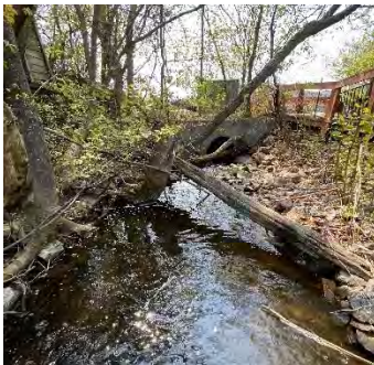
Description: Looking d/s
