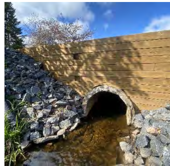
Description: Looking at d/s face
