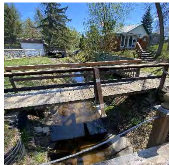
Description: Looking at d/s face
