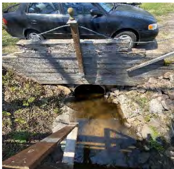
Description: Looking d/s
