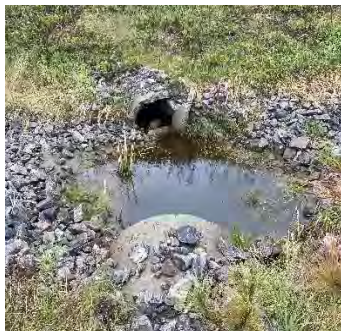
Description: Looking d/s
