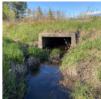
Description: Looking at d/s face
