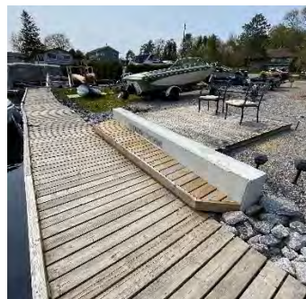
Description: Looking at d/s face
