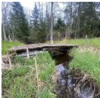
Description: Looking at d/s face
