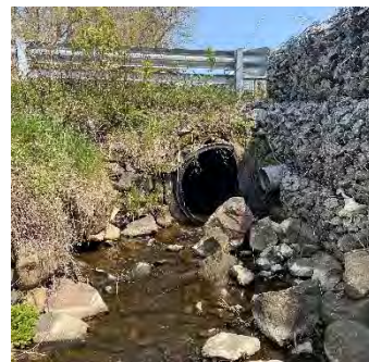
Description: Looking at d/s face
