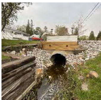
Description: Looking at d/s face
