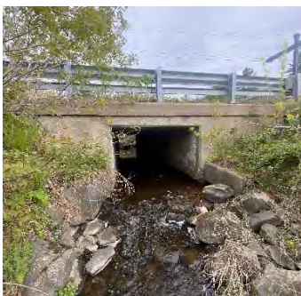
Description: Looking at d/s face
