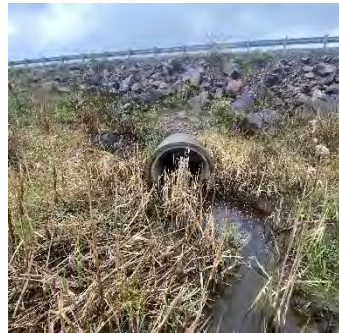
Description: Looking at u/s face
