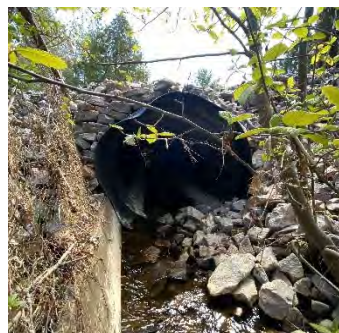
Description: Looking at d/s face
