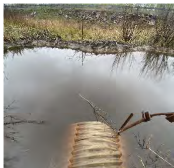
Description: Looking d/s
