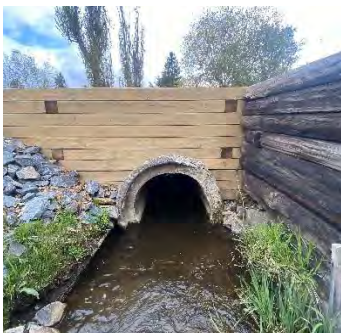
Description: Looking d/s
