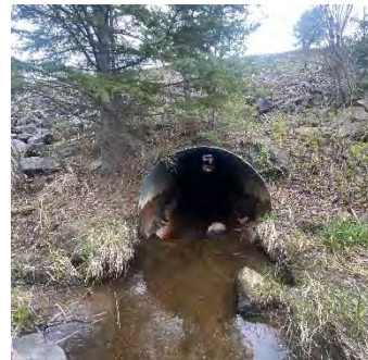
Description: Looking at d/s face
