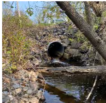
Description: Looking at d/s face
