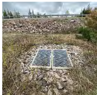
Description: Looking at d/s face
