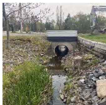
Description: Looking at u/s face
