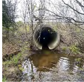
Description: Looking at u/s face
