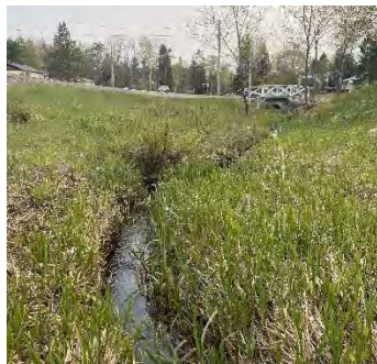
Description: Looking d/s
