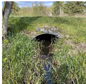
Description: Looking at d/s face
