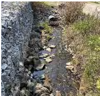
Description: Looking d/s
