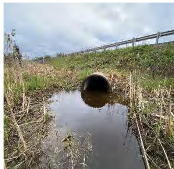
Description: Looking at d/s face
