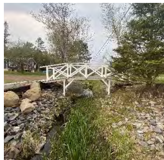
Description: Looking at d/s face
