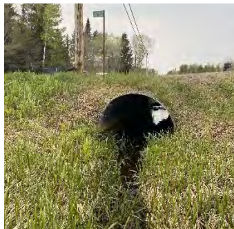
Description: Looking at d/s face
