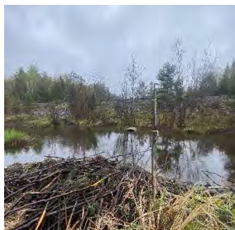
Description: Looking at d/s face
