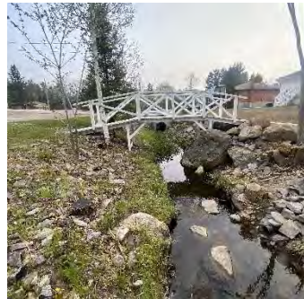
Description: Looking at u/s face
