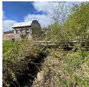
Description: Looking at u/s face
