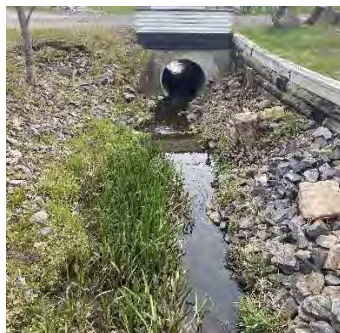
Description: Looking d/s
