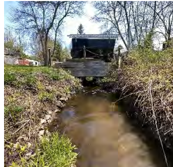
Description: Looking at d/s face
