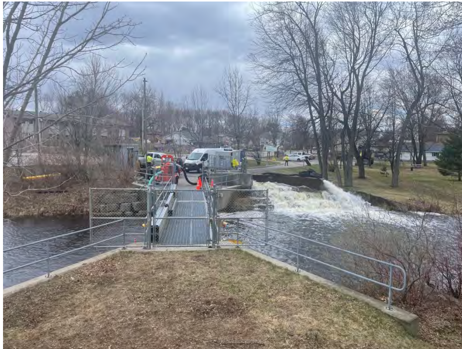
Figure 1 - Parks Creek Back Flood Control Structure
