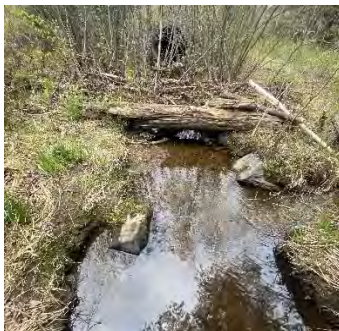
Description: Looking d/s
