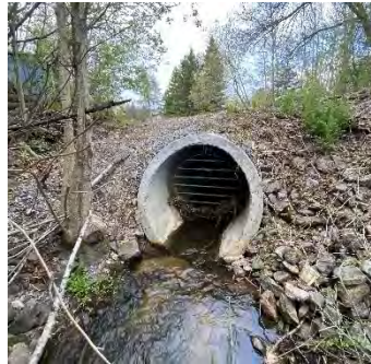
Description: Looking at d/s face
