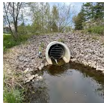
Description: Looking at d/s face
