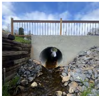
Description: Looking at d/s face
