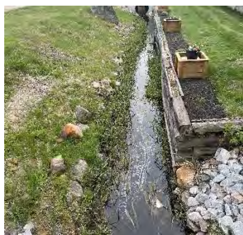
Description: Looking d/s
