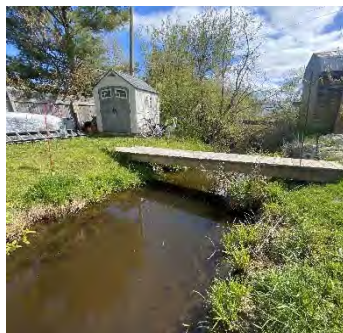
Description: Looking at d/s face
