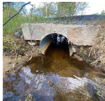
Description: Looking at d/s face
