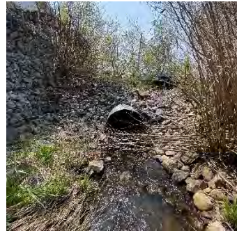
Description: Looking at u/s face
