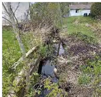
Description: Looking d/s
