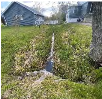
Description: Looking d/s
