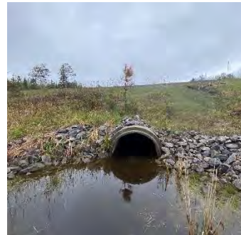
Description: Looking at d/s face
