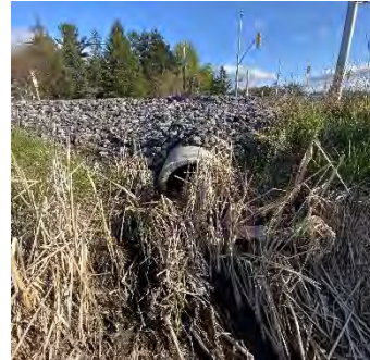
Description: Looking at d/s face
