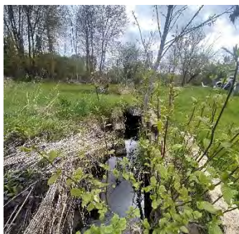
Description: Looking at d/s face
