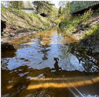
Description: Looking u/s
